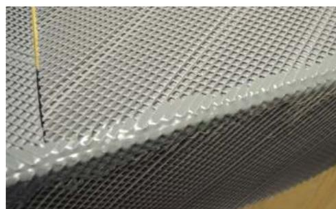
**2mm x 60mm seam of Polyurea WCS gun grade using large diameter static mixer (gunned similar style to a sealant) with manual gun. Excellent seam join between 2 adjoining strips of Proofex Engage.**
