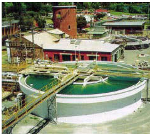
Nitocote EP405 applied to potable water tank at Shepparton
