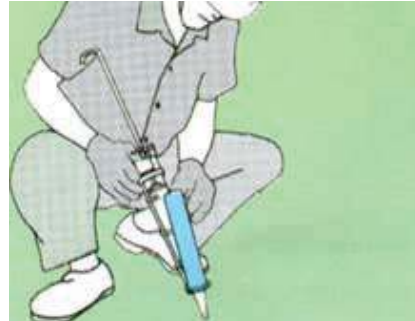
4. Set the cartridge to the caulking gun.
