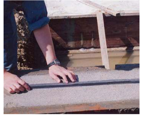
PLACE KUNISEAL ON JOINT AND PRESS IN PLACE.
