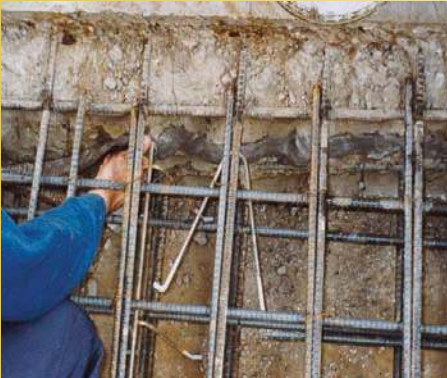
SLOWLY PRESS ON TO CONNECTING SLAB JOINT.
