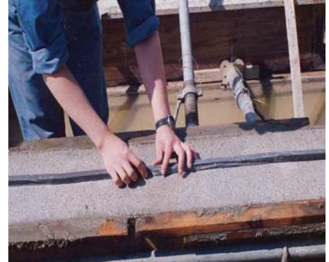
CONNECT TWO PIECES BY END-BUTT JOINING.
