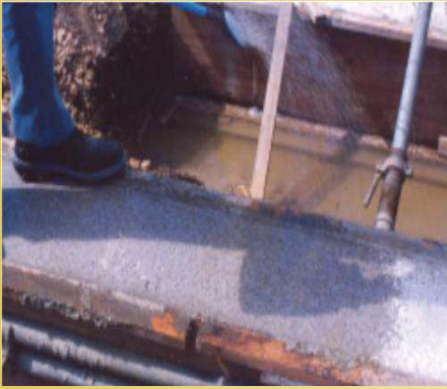
BRUSH OFF DIRT AND WET CONCRETE JOINT.
