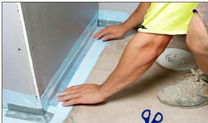
Installing Elastoproof B50 Bond Breaker Joint Band
