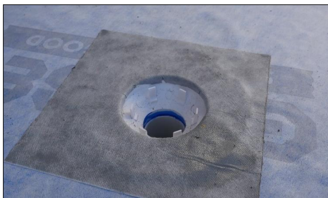
Elastoproof Butyl Square over leak control flange
