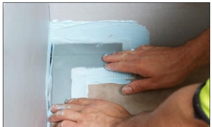
Installing Elastoproof Prefabricated Corners
