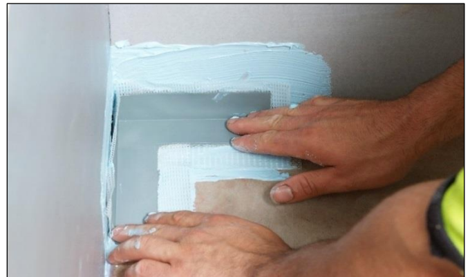
Installing Elastoproof Prefabricated Corners
