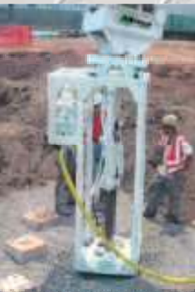
A-2SD Vertical Equipment mounted drill used for drilling on foundations
