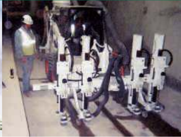
A-4SD Vertical Equipment mounted drill used in tunnel construction.
