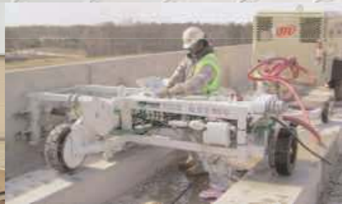
A-4SD Core Drill used for light rail construction.
