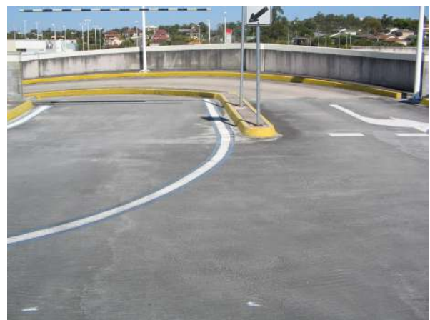
Rain damaged roof deck resurfaced with Aegis MSP
